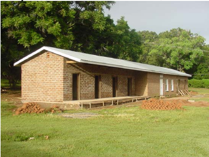
Chimala Mission library undergoing renovation with added offices and increased space.
